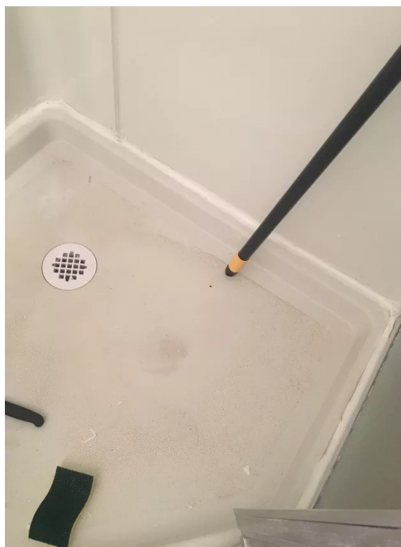
Low-cost shower surfaces can stain, dull, and become harder to make look clean over time.
