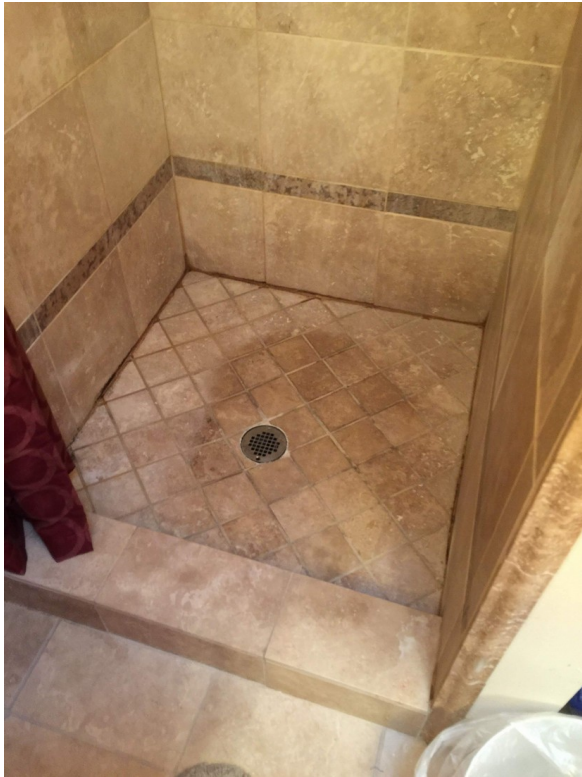
Tile can look beautiful, but grout lines and hard-water buildup become part of the maintenance burden.
