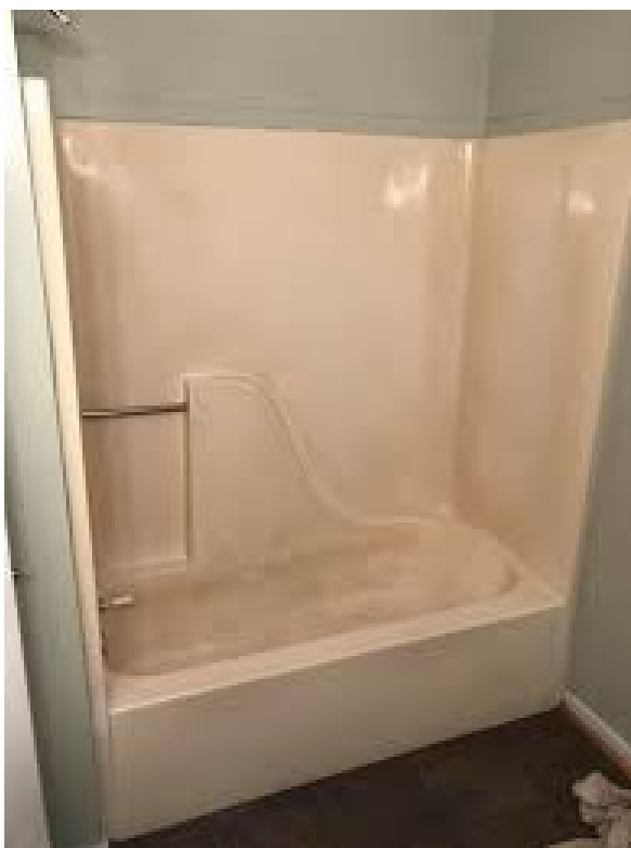
Example of an older fiberglass tub/shower that has yellowed and lost its clean appearance.
